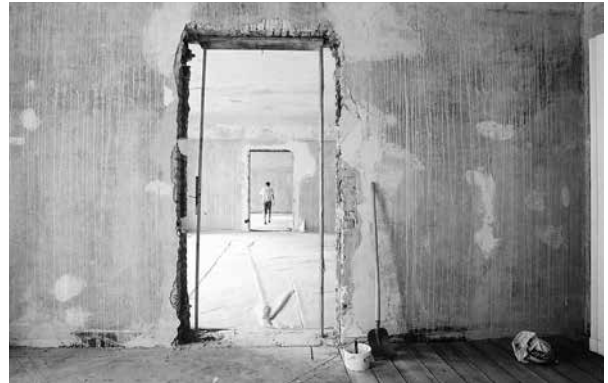
Renovation of the gallery Arndt & Partner, Checkpoint Charlie, Berlin, 2001
